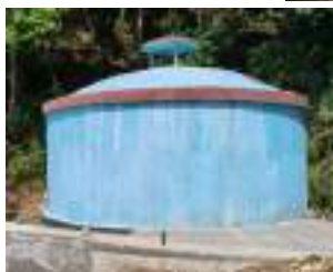
200cu.m,100cu.m RCC Ground Tank
