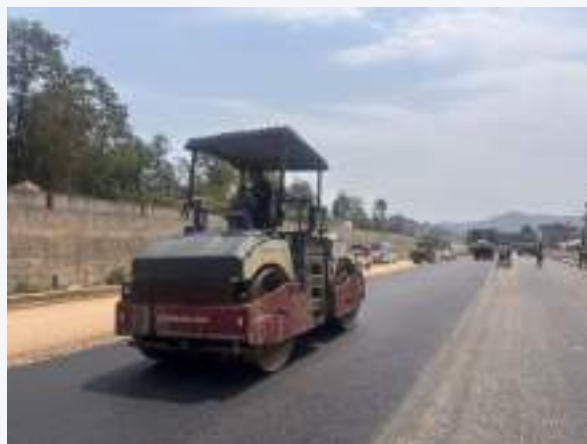
DBM WORKS (SANGA DHULIKHEL SECTION)
