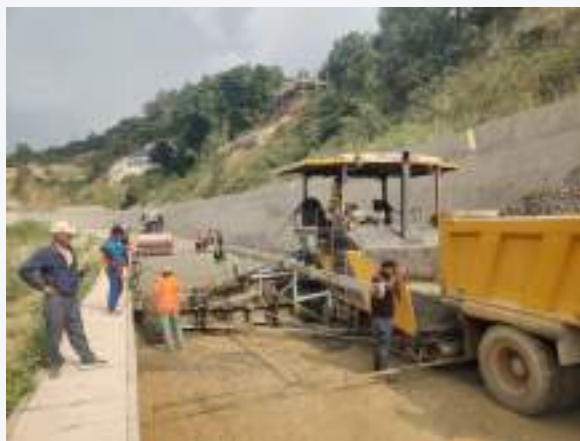
CTB WORKS AT SANGA (CHAINAGE 5+850-6+770)
