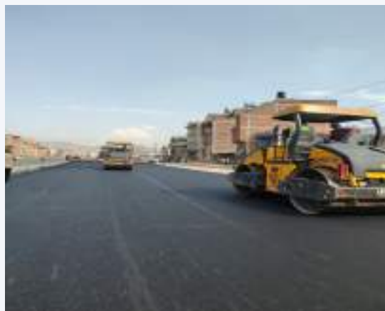
DBM WORKS AT SURYABINAYAK JAGATI SECTION ( CHAINAGE 0+060-1+575)
